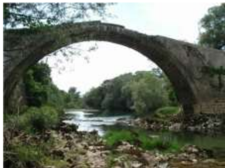
Figure 06. Bridge of the Klepci near Capljina (Photo: http://www.panoramio.com/photo/14435409 )
