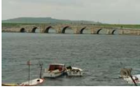
Figure 19. Sultan Suleiman the bridge, Büyükçekmece, Turkey (1568)
