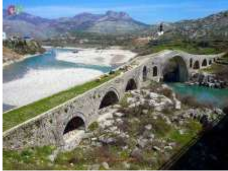
Figure 25. Mes Bridge (Ura e Mesita) on the Kir river, near Shkoder, Albania (1770)
