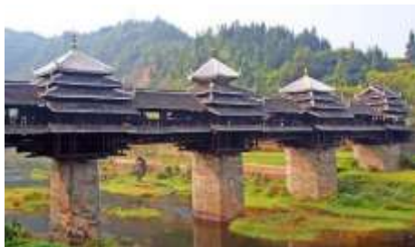
Figure 05. Chengyang Bridge, China (1912)
