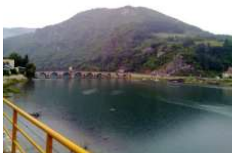
Figure 12. Mehmed Pasha Sokolovoća Bridge in Visegrad (Photos: Prof. dr A. Hadrović, 04.08.2011.)
