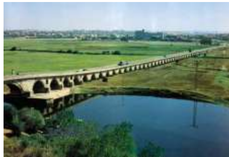
Figure 18. Long Bridge (Uzunköprü) on the Ergen river, Uzunköprü near Edirne (1426-1443)
