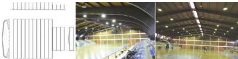
Figure 15. Large span glulam timber structure, Vushtrri
