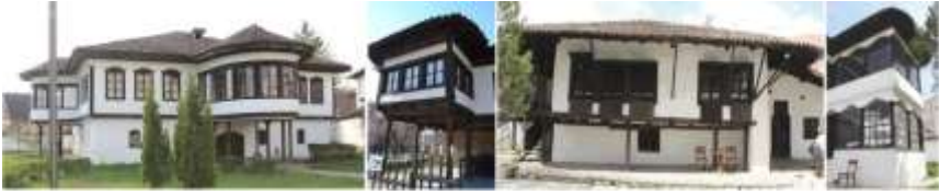
Figure 2. Combined structure house Kosovo
